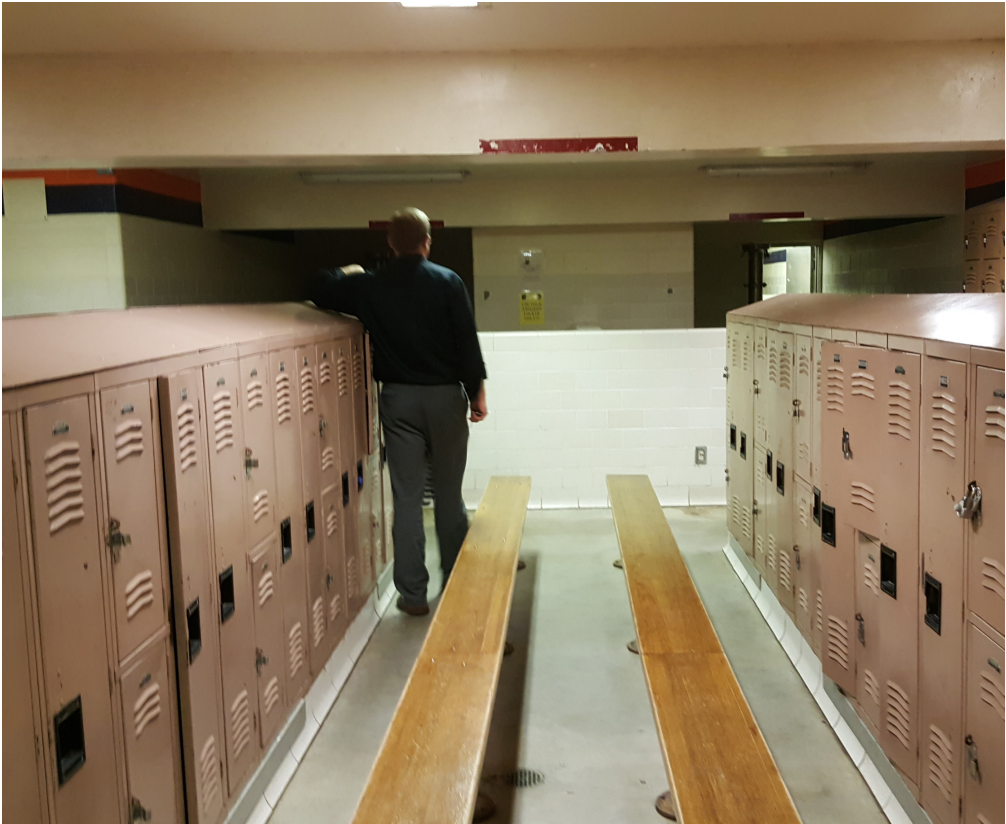
Existing locker facilities, the existing ceiling height cannot accommodate new duct work.
